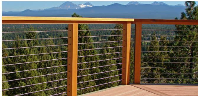
Wood cable system with Threaded Receiver (no visible fittings)
